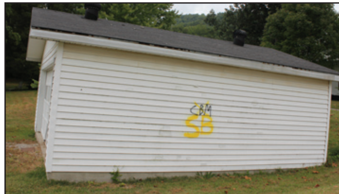
Over the last several weeks vandals have been spray painting graffiti on buildings in Hudson, George, High and Cantrill Streets in Irvine. The garage above has CBM spray painted in black. Then it was sprayed with a yellow X over the black and the initials SB below it. Residents who see any suspicious activity are asked to call the non-emergency dispatch number at 723-2201.
