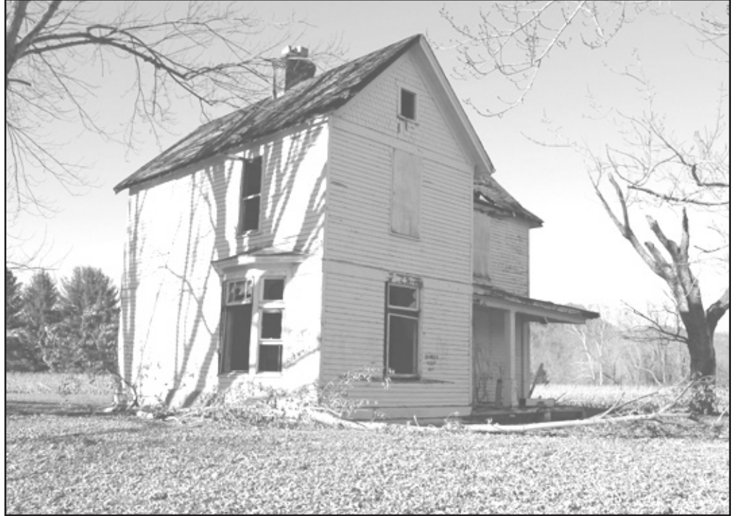
Two lock houses remain standing at Lock 12 but are in a bad shape of disrepair. Local leaders once wanted to make a museum of one of the lock houses. Thursday's conference has renewed local interest into restoring the beaches at Lock 12 and making the area into a park.
