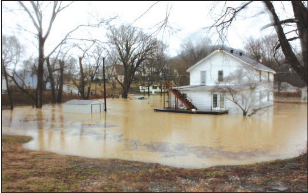
This photo taken from River Drive shows water surrounding a house on Main Street of Ravenna near the Irvine city line.
