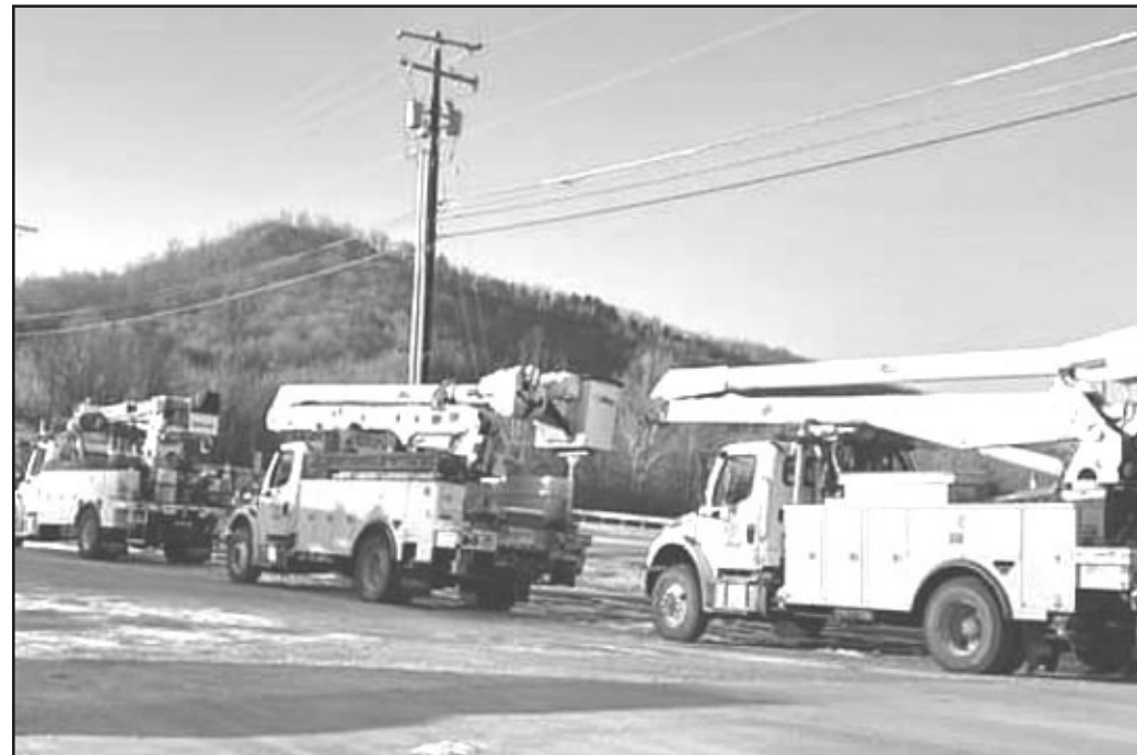
Electricity has been restored to most Estill County customers of Jackson Energy as of Tuesday morning, but contractors and other energy cooperatives remained in the area until all power is restored. The trucks above were lined up on the Winchester Road Tuesday.
