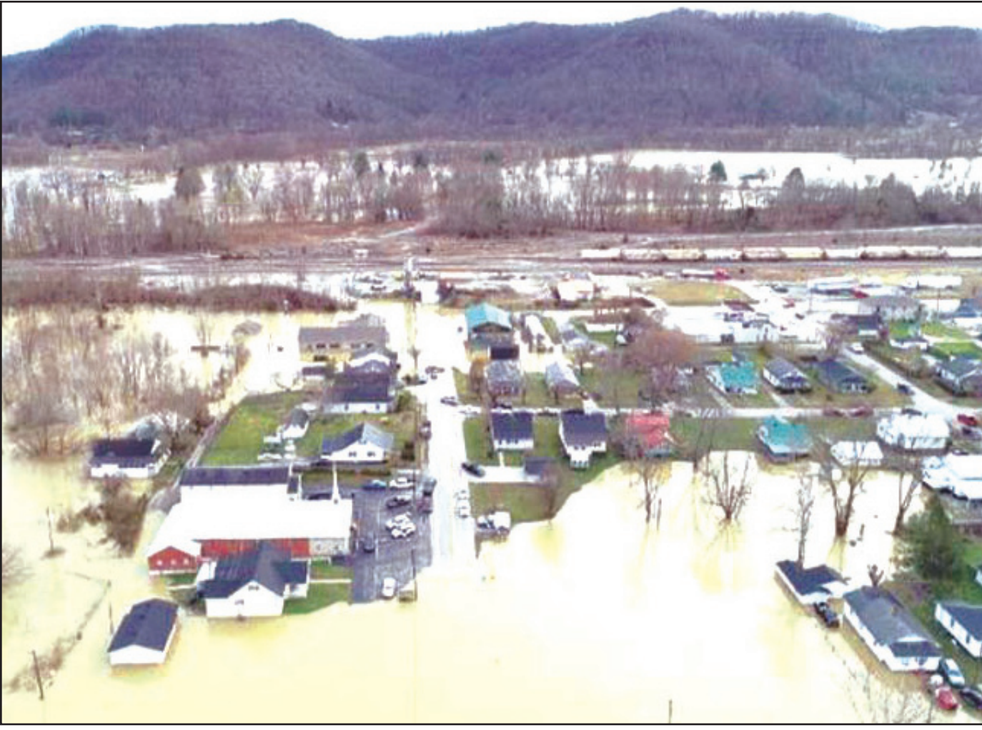
This photo was shared on Facebook of Third Street in Ravenna, also known as KY 52. The Ravenna Church of God is in the front left. Michael's Restaurant on the corner was originally scheduled to reopen Thursday.
