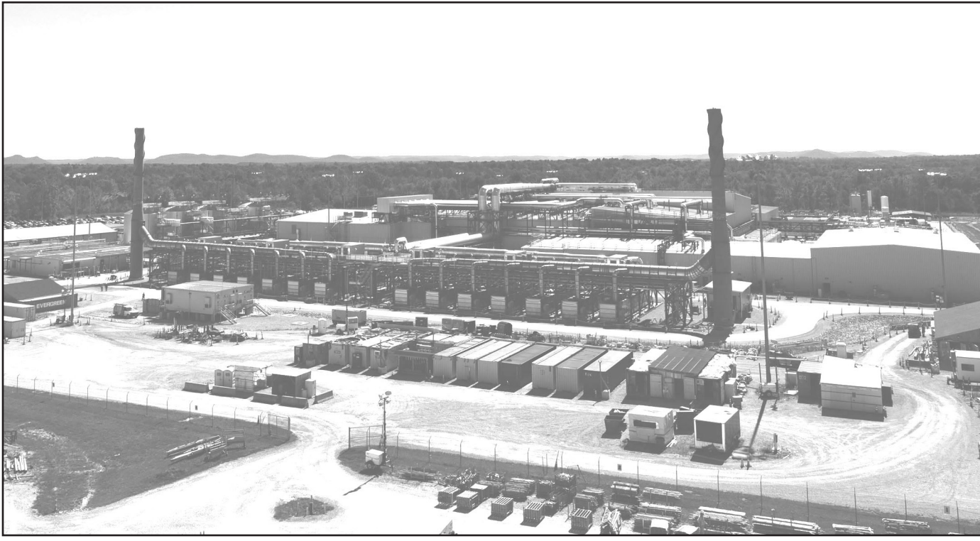
An aerial view of the finished Chemical Weapons Facility
