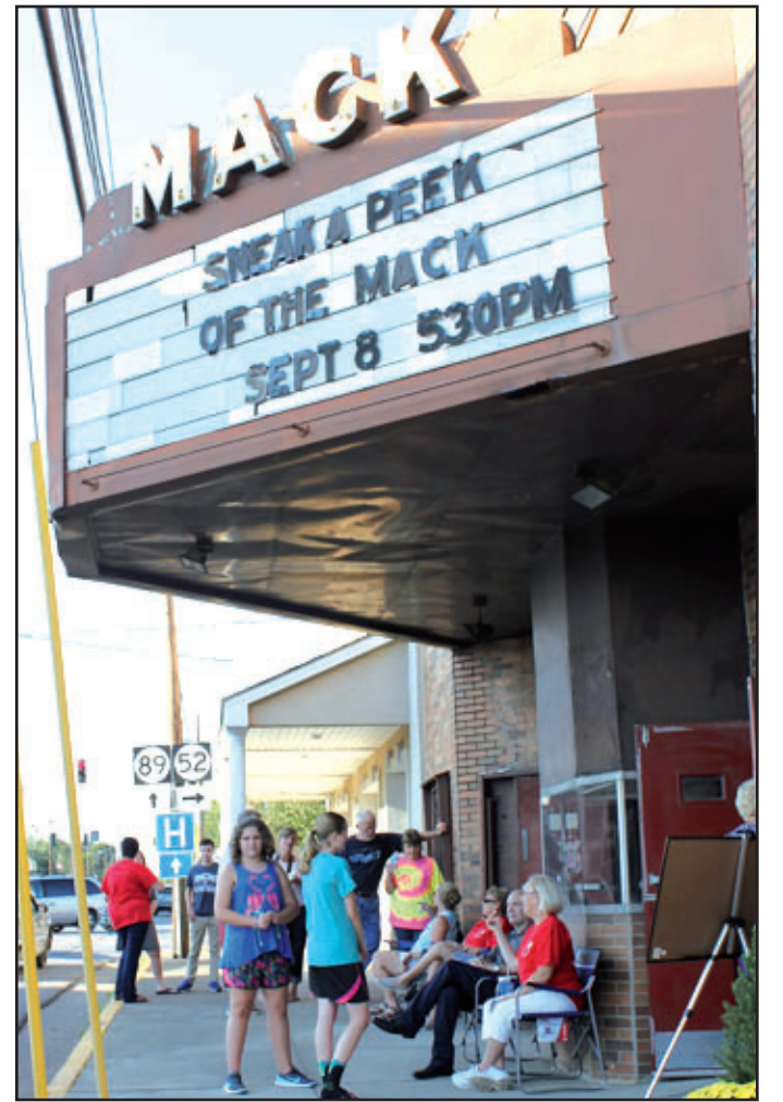
The River City Players purchased the Mack Theatre building in 2016, applied for a brownfields grant and received it for $200,000 to clean up lead paint and asbestos. File Photo
