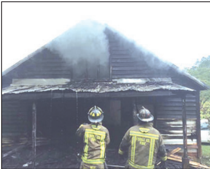
Estill County Firefighters Chad Neal and Shawn Riddell look at a house which burned Monday morning on Mt. Zion Road. The family living in the home lost everything. The cause of this fire and the one Saturday are not being considered as suspicious. Photo courtesy of Estill Co. Fire Dept.
