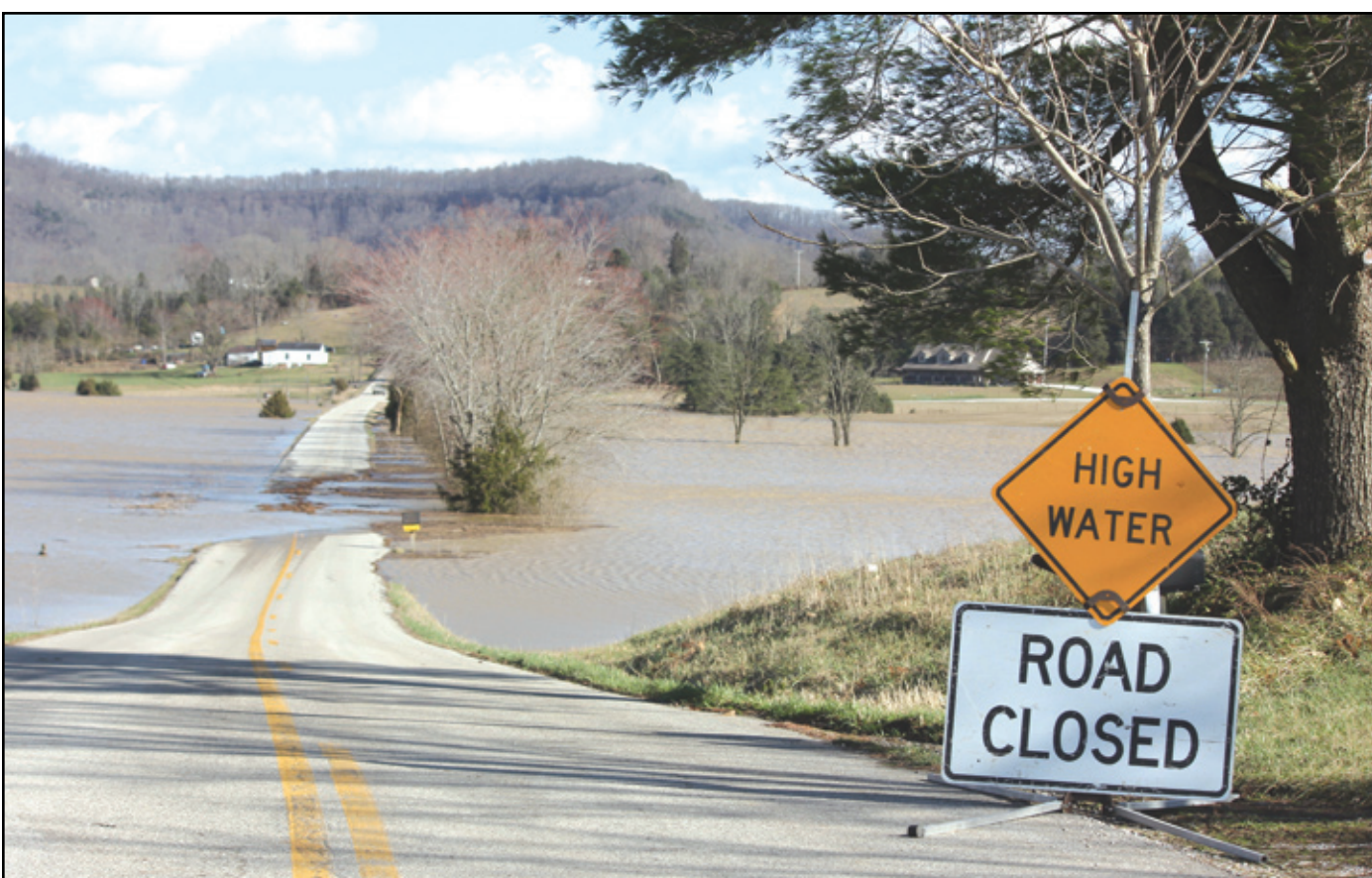
Water had started to cover Maupin Hill Road Sunday afternoon. Most vehicles chose not to travel through the water. High winds were creating large waves in the flood waters.
