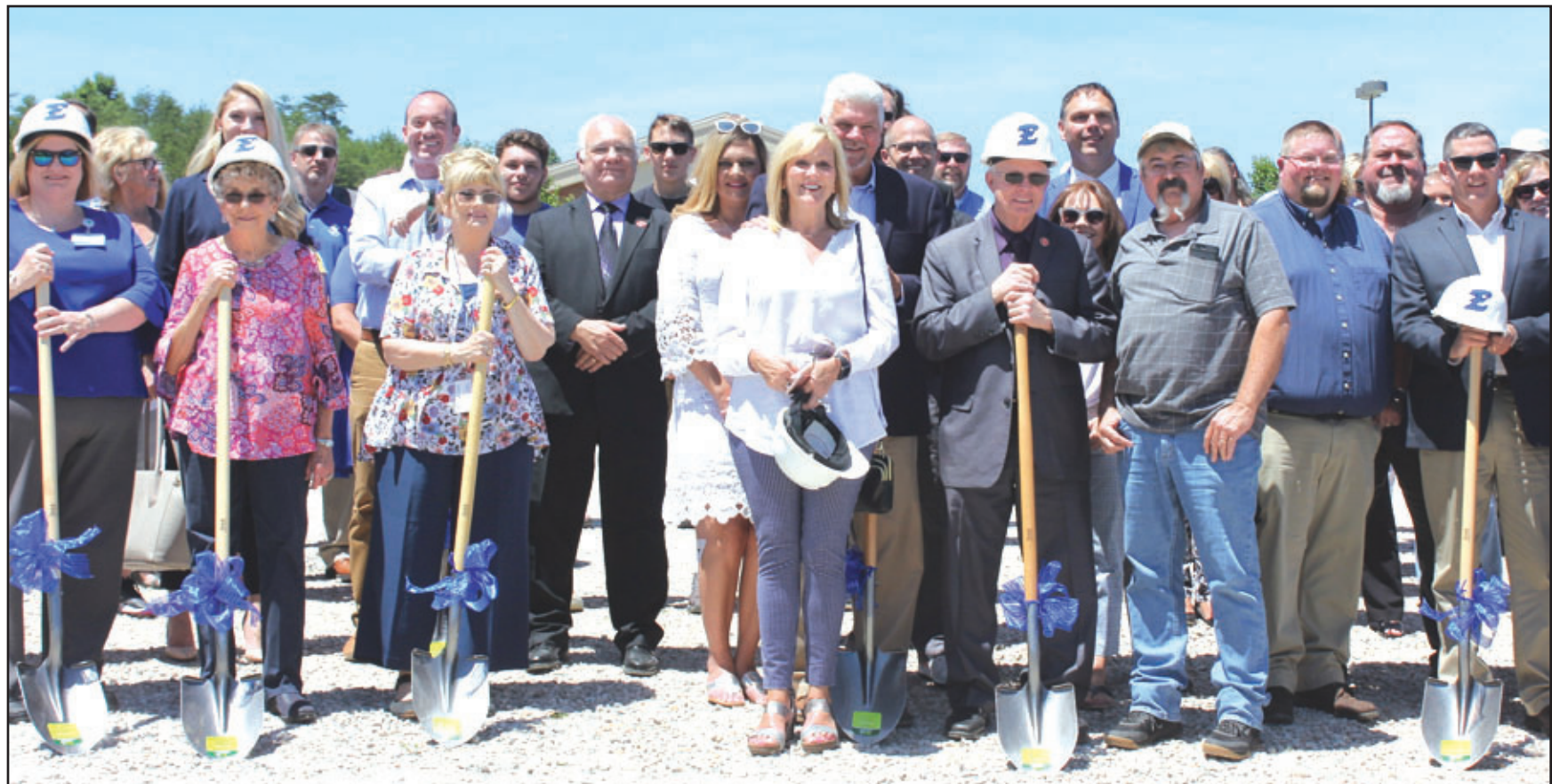
Groundbreaking for Estill County's new Area Technical Center (ATC) was held on Friday afternoon. Different groups got involved with breaking the ground in the gravel parking lot where the school bus garage is now located. Above, nearly everyone got into the act. Less than half those present are pictured in the photo above.
